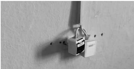
Damaged socket at Ig Prison
