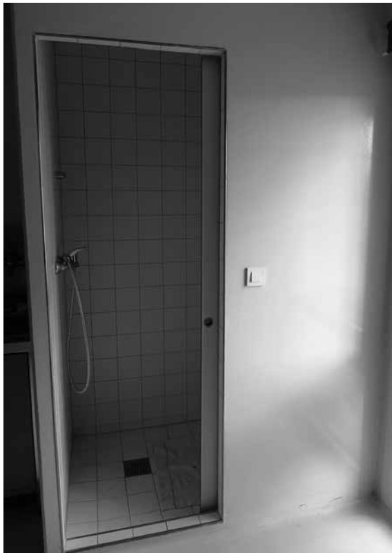
Bathroom and toilet in the hospital room in Department V of Dob Prison with a narrow entrance, high doorstep and no grab bars.
